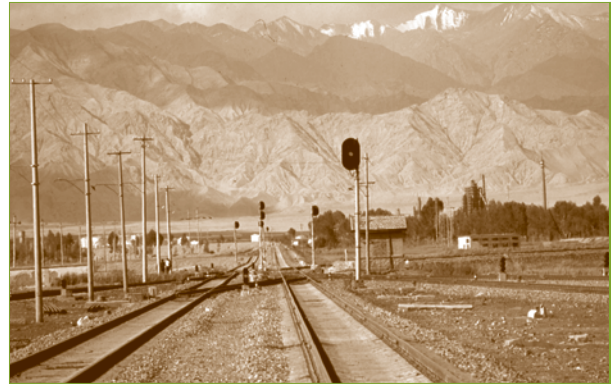
Beyond Gormo, the rail line will climb over the 16,641 ft (5,072 m) Tanggula pass and will require an estimated 286 new bridges. (Photo: ICT)
