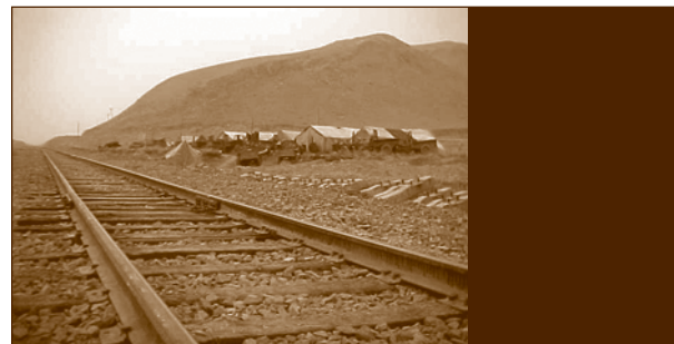
This camp south of Gormo is a temporary construction camp, but many new permanent settlements will be built for maintenance workers, signal stations and sidings. (Photo: ICT)
